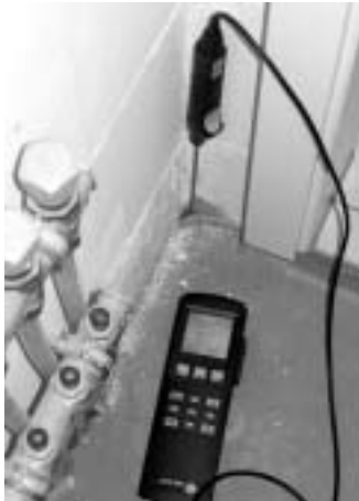
Abb. 7: Messung in Estrich-Randfuge
